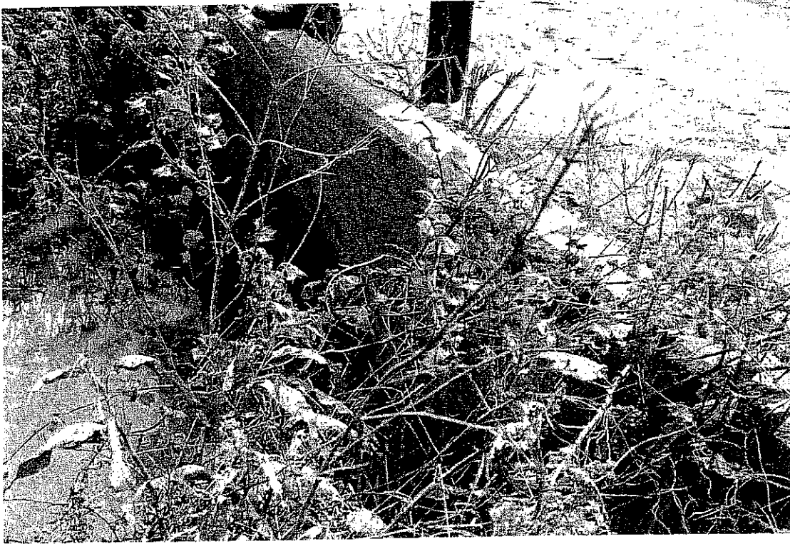
Above & Below - Cement bridge built by Wm. H. Bockhaus in 1911 - still in use in 1995 along the county road that leads to the old home place near Halstead, Ks.
